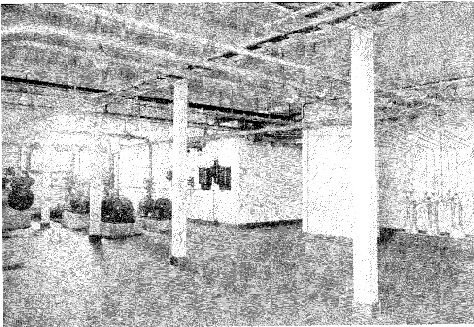
Figure 4—The Basement at Kalundborg.
