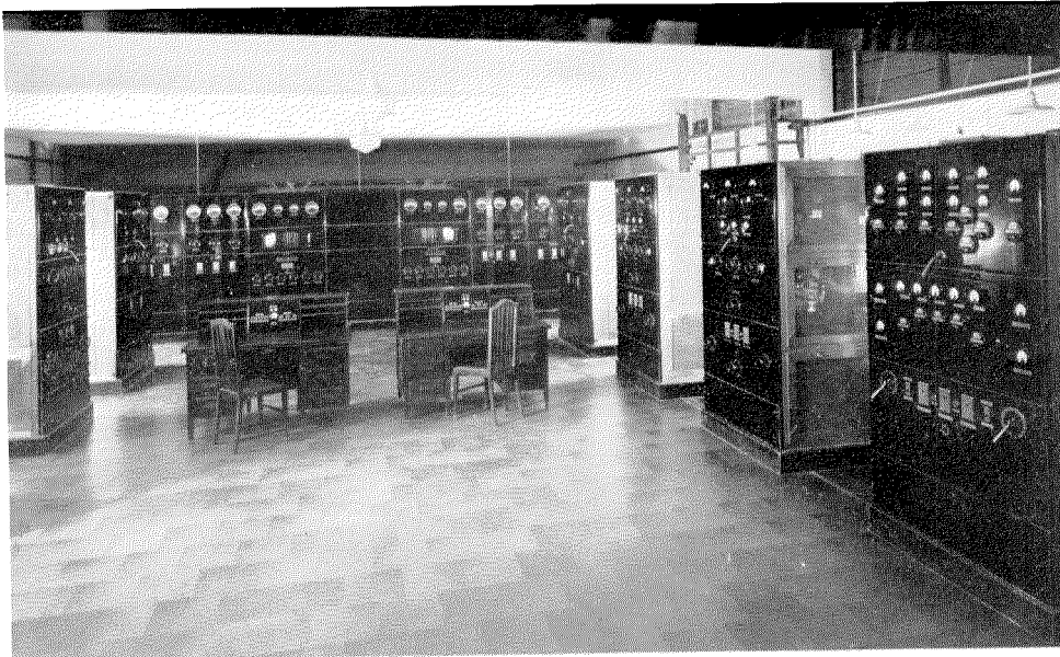
Figure 5—Transmitter Hall Showing Twin Transmitters on Either Side and Power Control Board at End.
