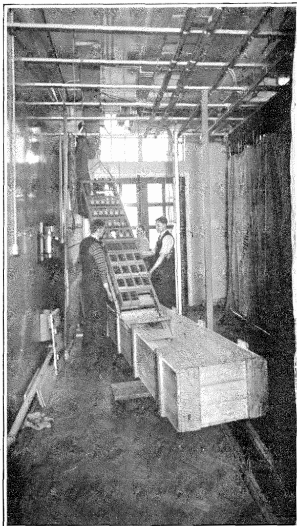
Figure 2—Penultimate Bays Being Raised from Case.
